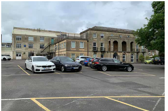
Avon House and mid 20 th century extension to west
